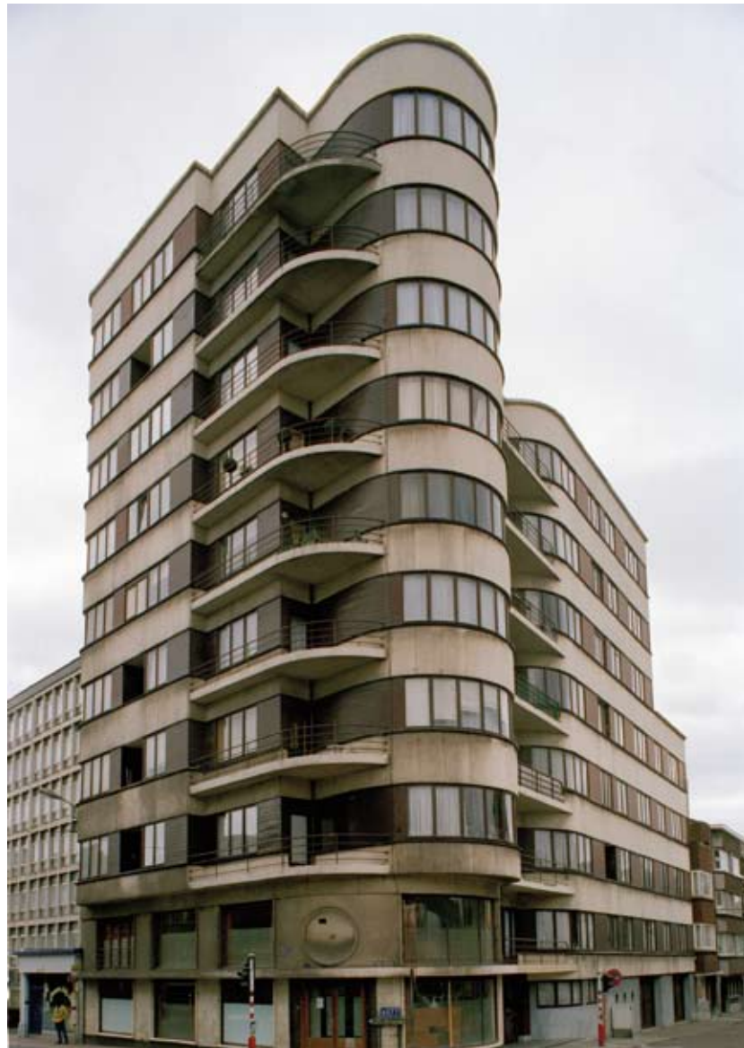
Photo F. Dor © SPW-DGATLPE
